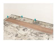
2. INSTALL FIRST PLANK Position the first plank against a spacer a few millimeters from the starting wall.
